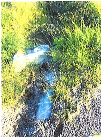
Above: Inadequate swales with crushed tin horn along 49 th on September 17, 2019
