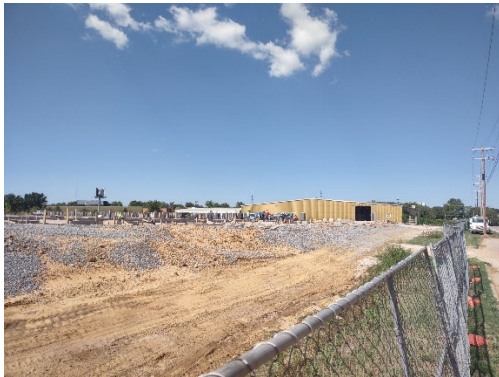
Allied Stone Expansion in progress
