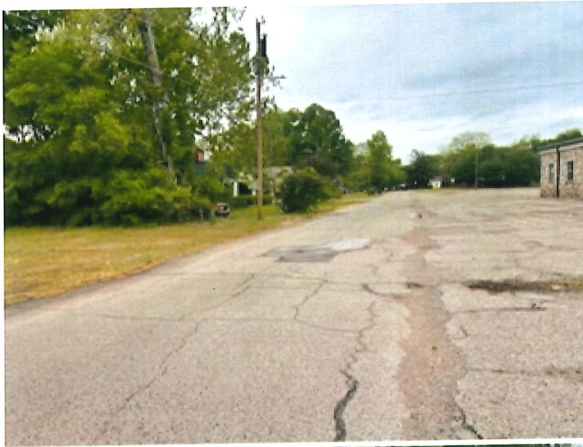
WEST STREET VIEW
