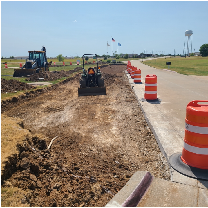
Right Side West Parking Lot
