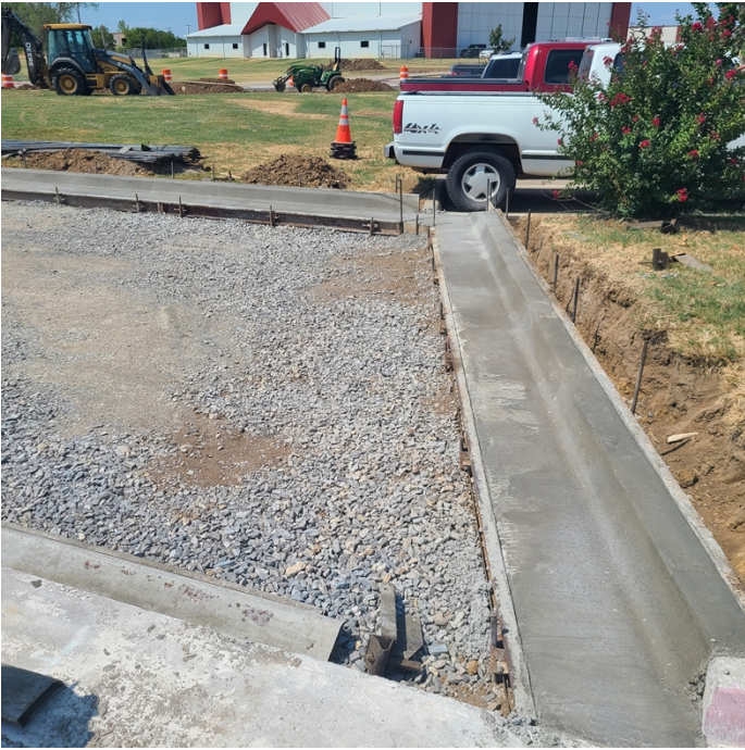
Left Side Curb West Parking Lot.
