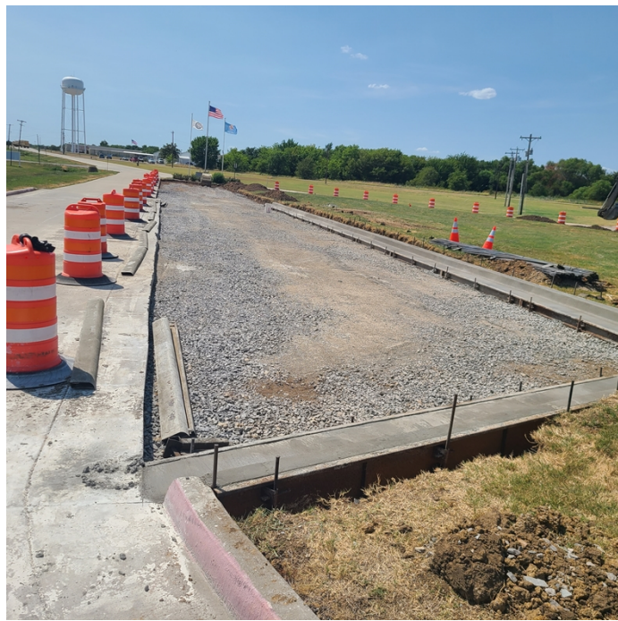
Left Side West Parking Lot
