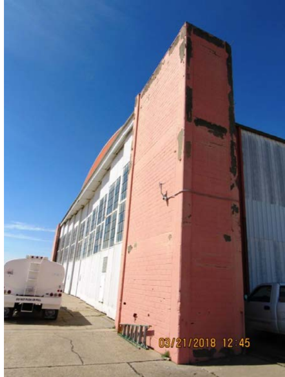
Exterior Area of the Site Abutting Southeast Door System
