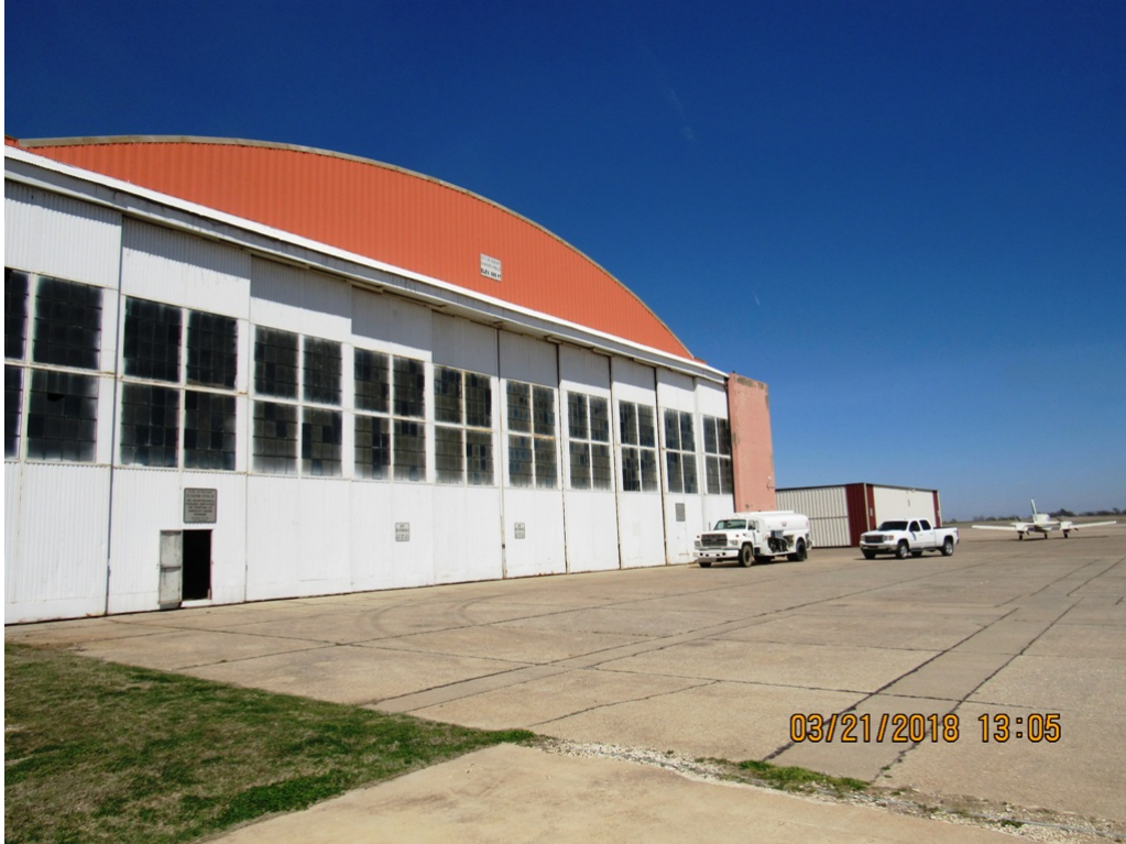
View of the Apron Portion of the Site on the Southeast Side of the Hangar
