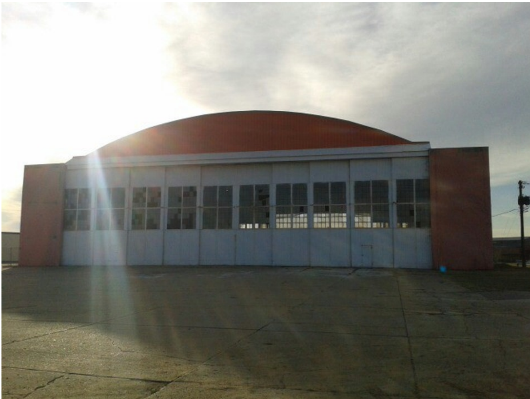
View Of The Northwest Hangar Door From The Ramp
