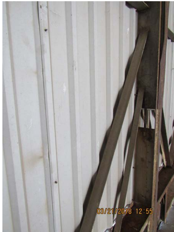
Close-Up of Hangar Door Frame
