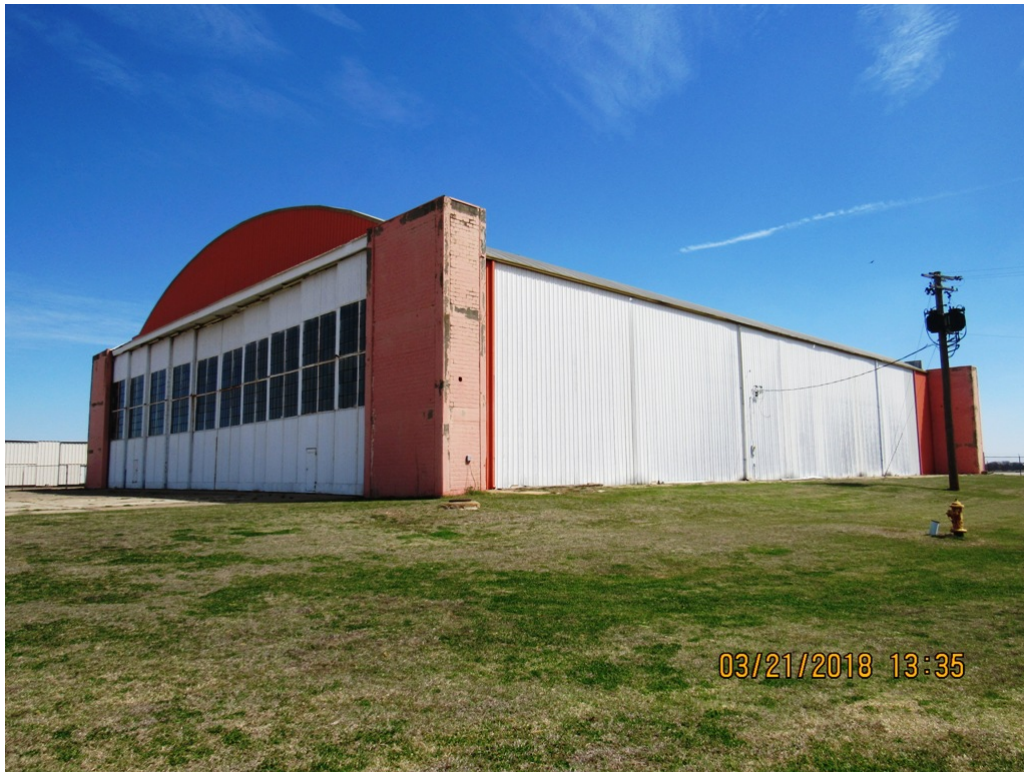
View of the Site from Approximately the South
