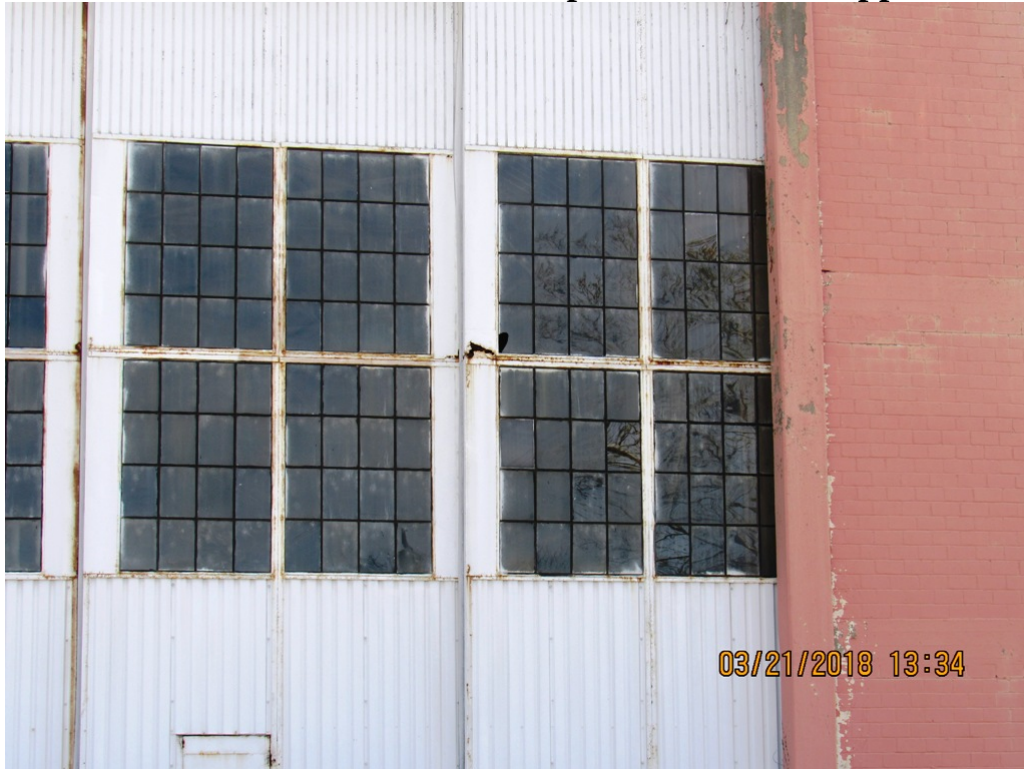
View Of Hangar Door And Door Pocket Interface
