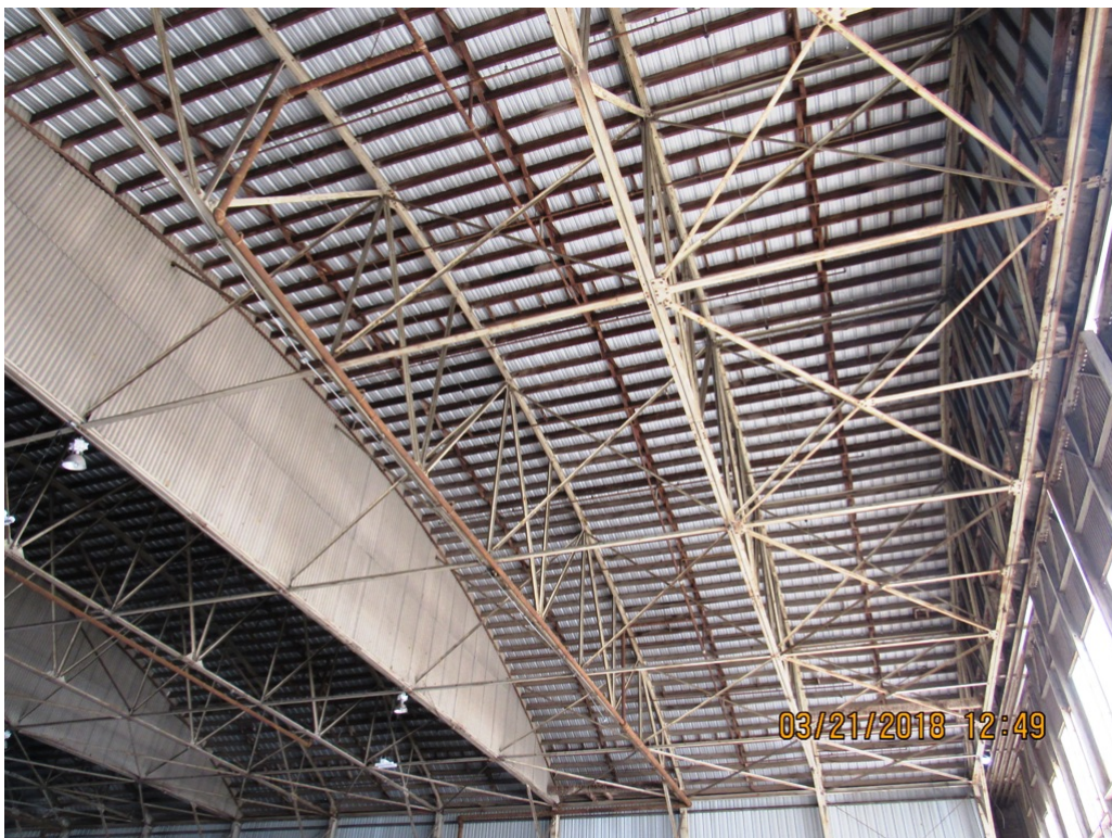
Interior View Of Hangar Roof Truss System
