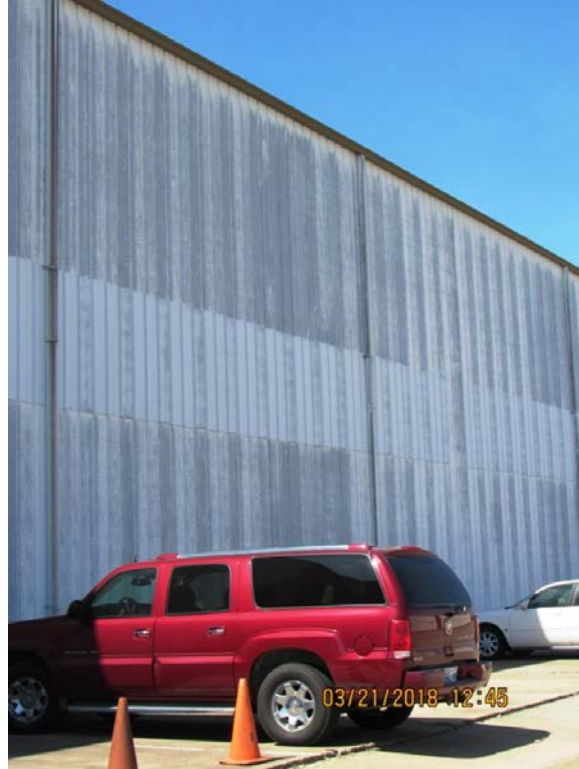
External View of Northeast Wall System
