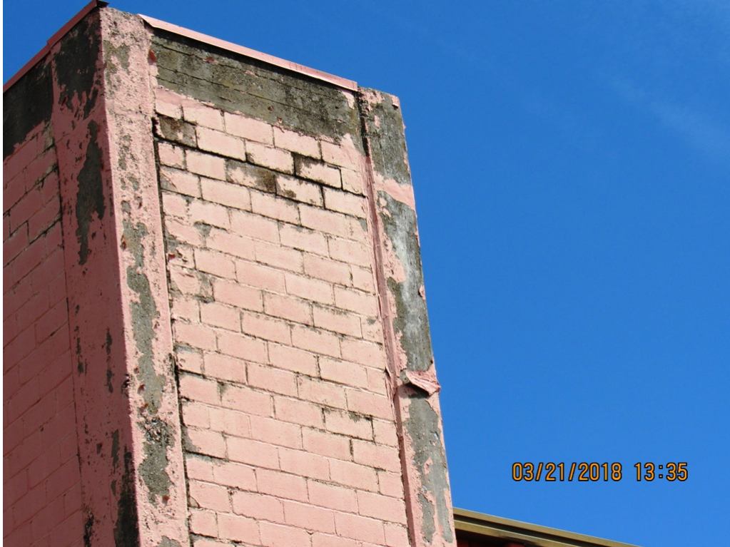
View Of Exterior Door Pocket Showing Brick and Block Condition
