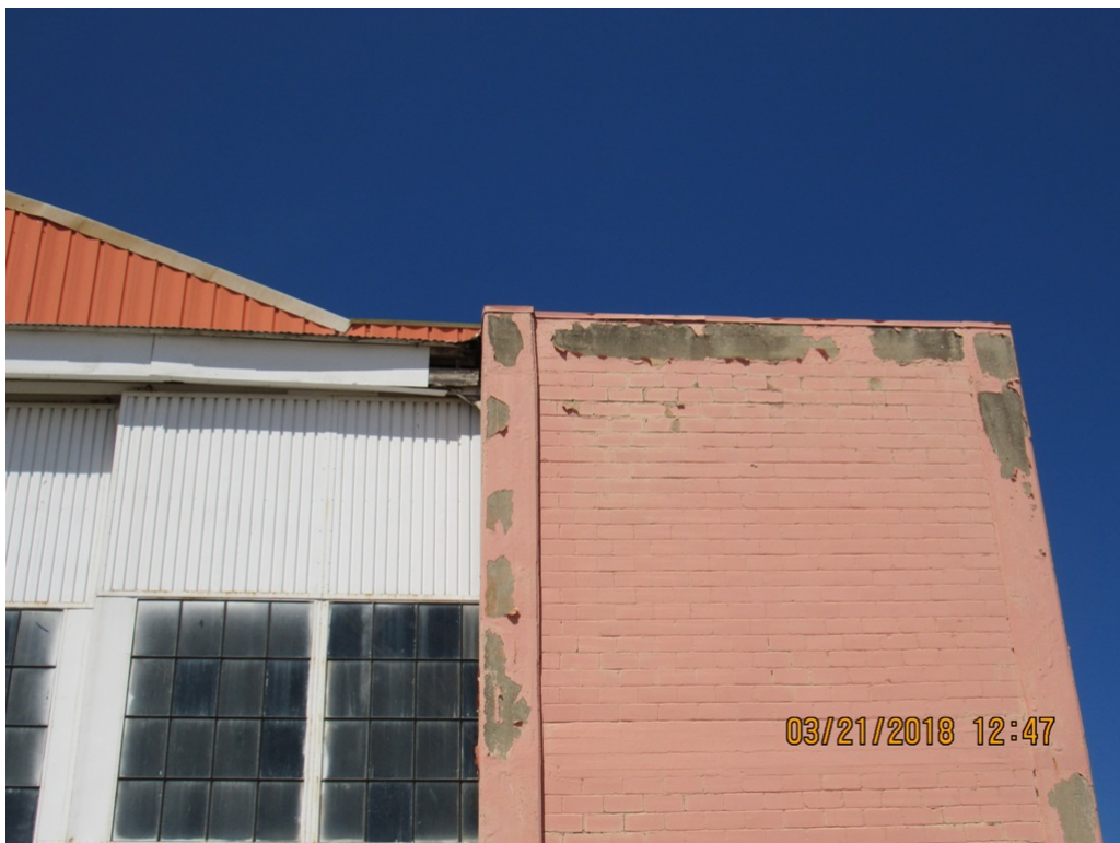
Exterior View of Upper-Level of Door Pocket
