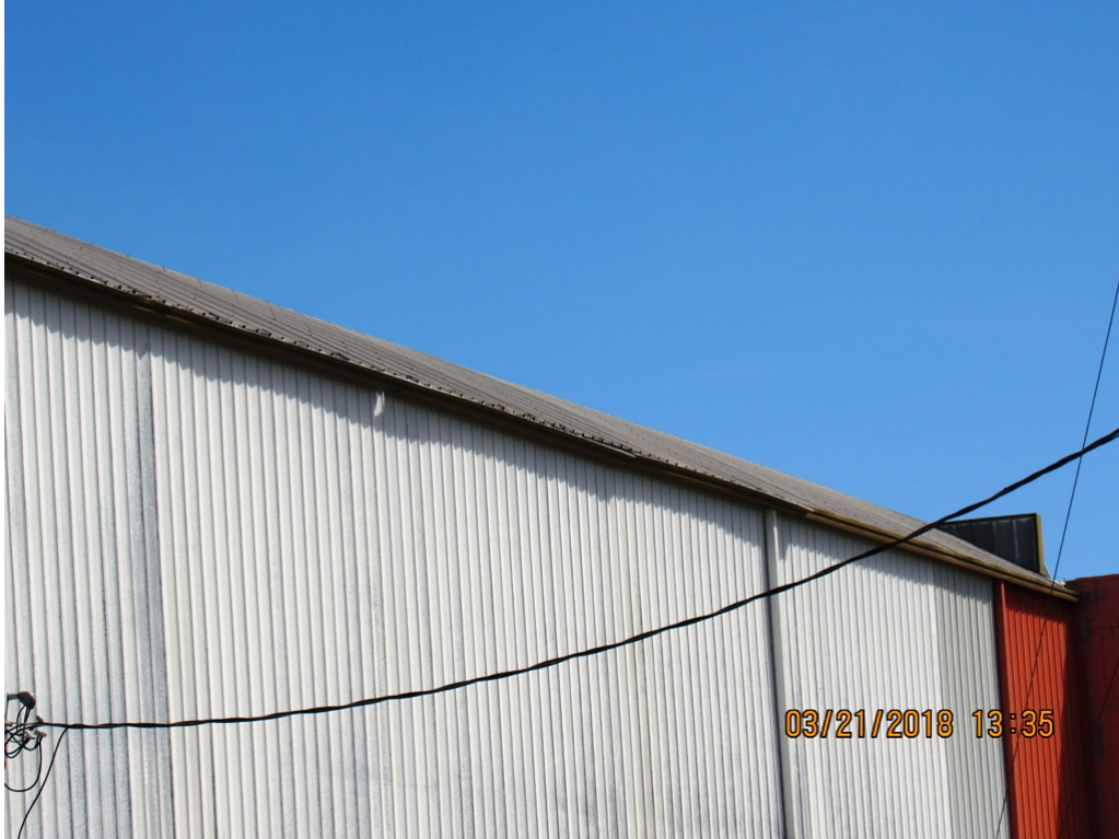
External View Of Galvanized Paneling With Baked -On Enamel Finish On Wall
