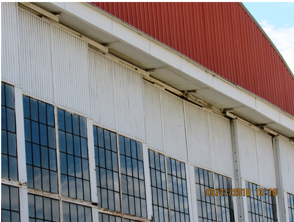
Upper-Level Door Tracks From The Outside
