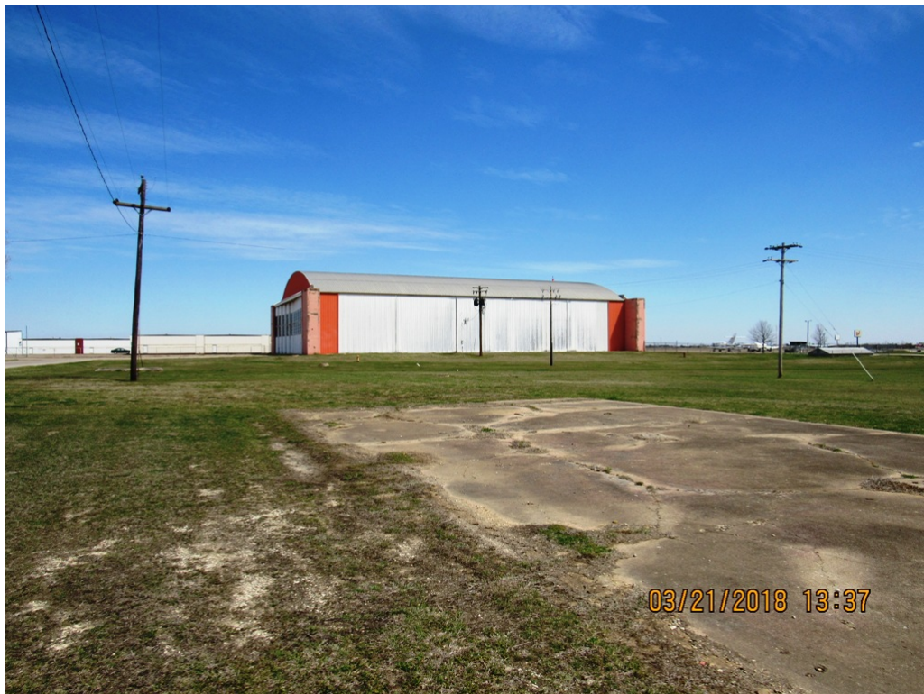
View of the Site from the General Area of the Terminal Building
