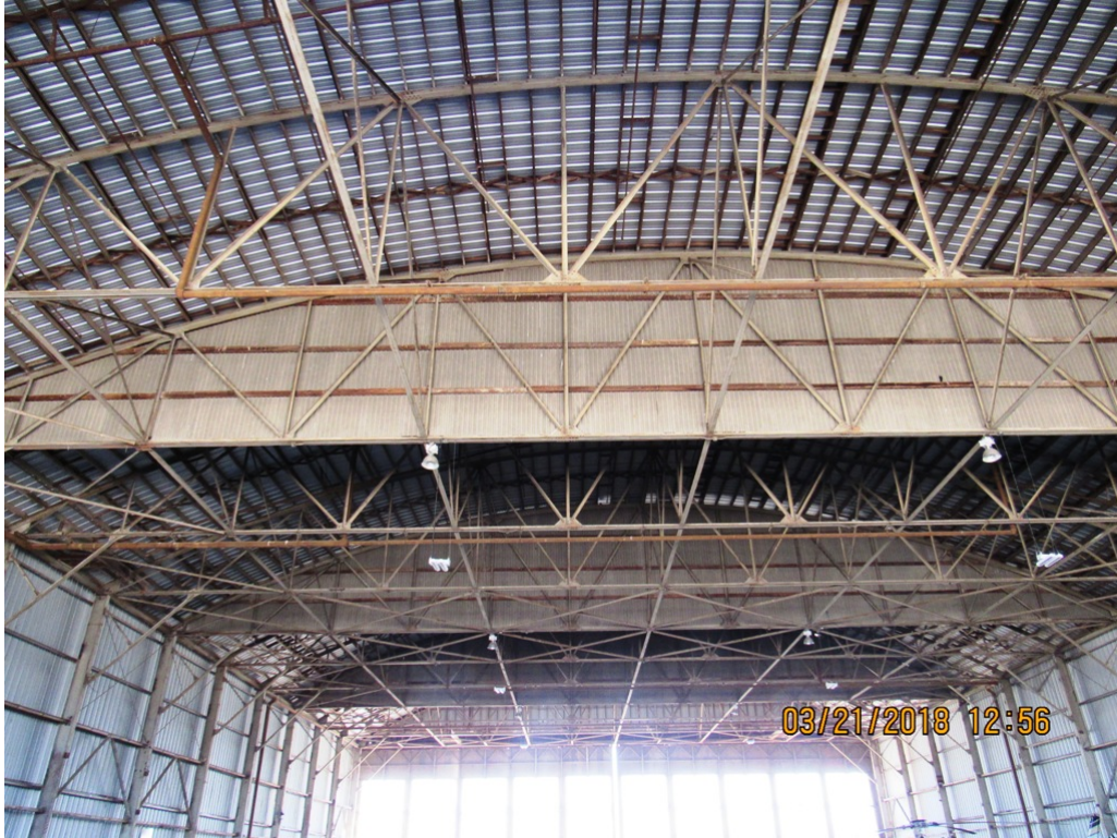
View of the Underside of the Hangar Roof System
