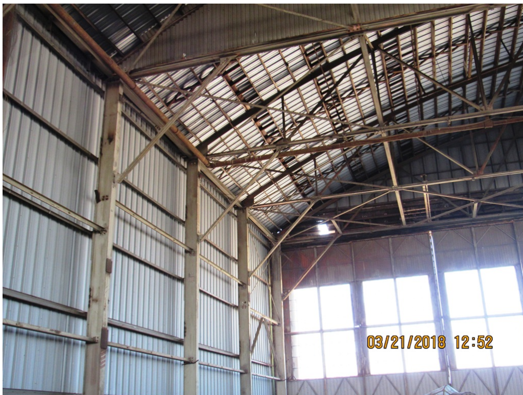
Interior View Showing Vertical Support Members
