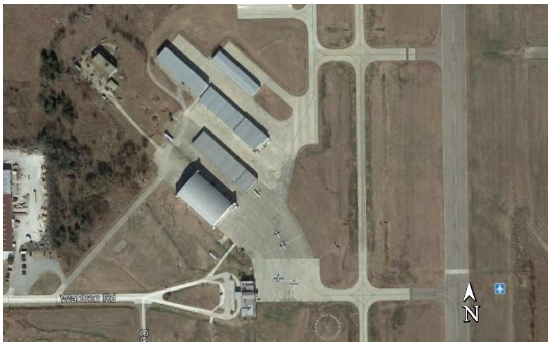
General Location Of The Subject Property On The Northwest Portion of the Airport
