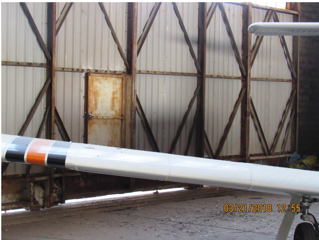
Interior View of Hangar Personnel Door
