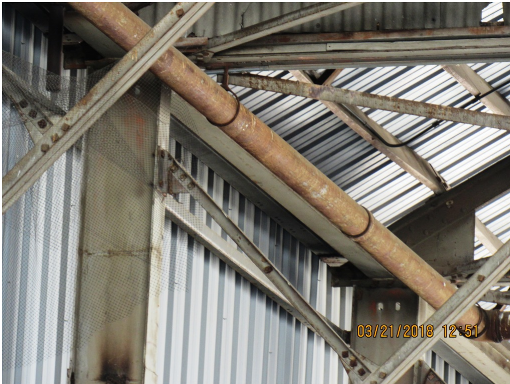
View of Piping Which Was Previously Installed to Support a Sprinkler System
