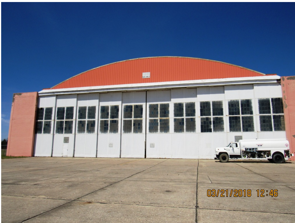
Area of the Site Adjacent to the Southeast Door System
