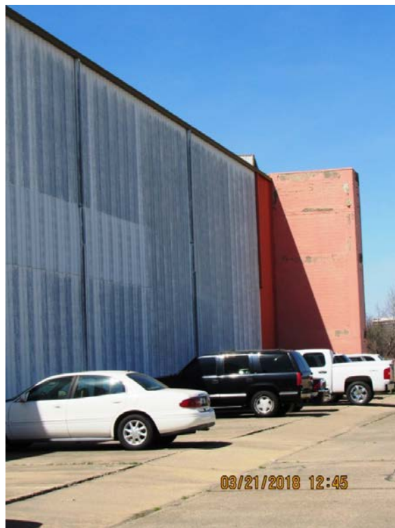
Paved Area Adjacent to the Northeast Hangar Wall
