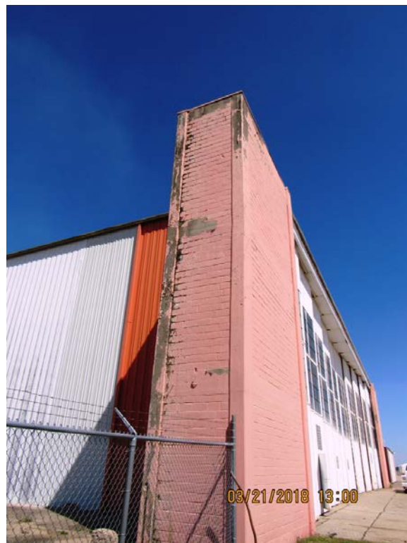
View Of Block And Brick Door Pocket
