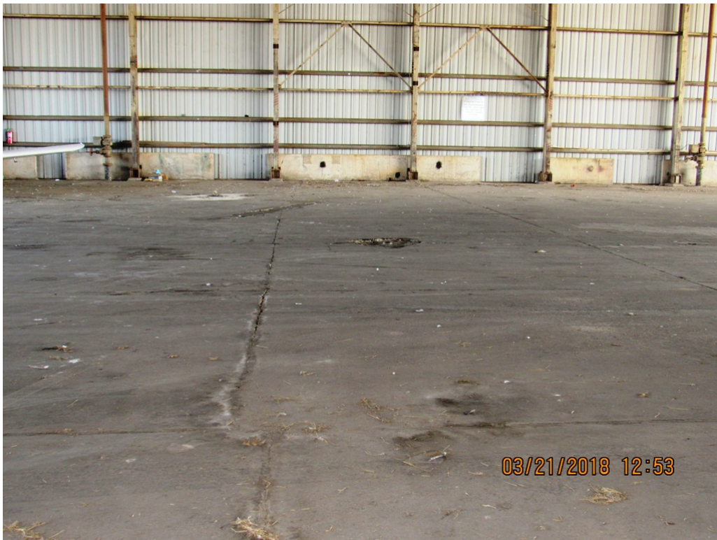
Interior View Of The Hangar Floor System
