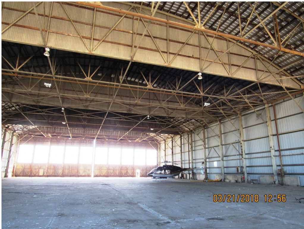
Interior View Of The Hangar Looking Toward The Northwest Door System Area
