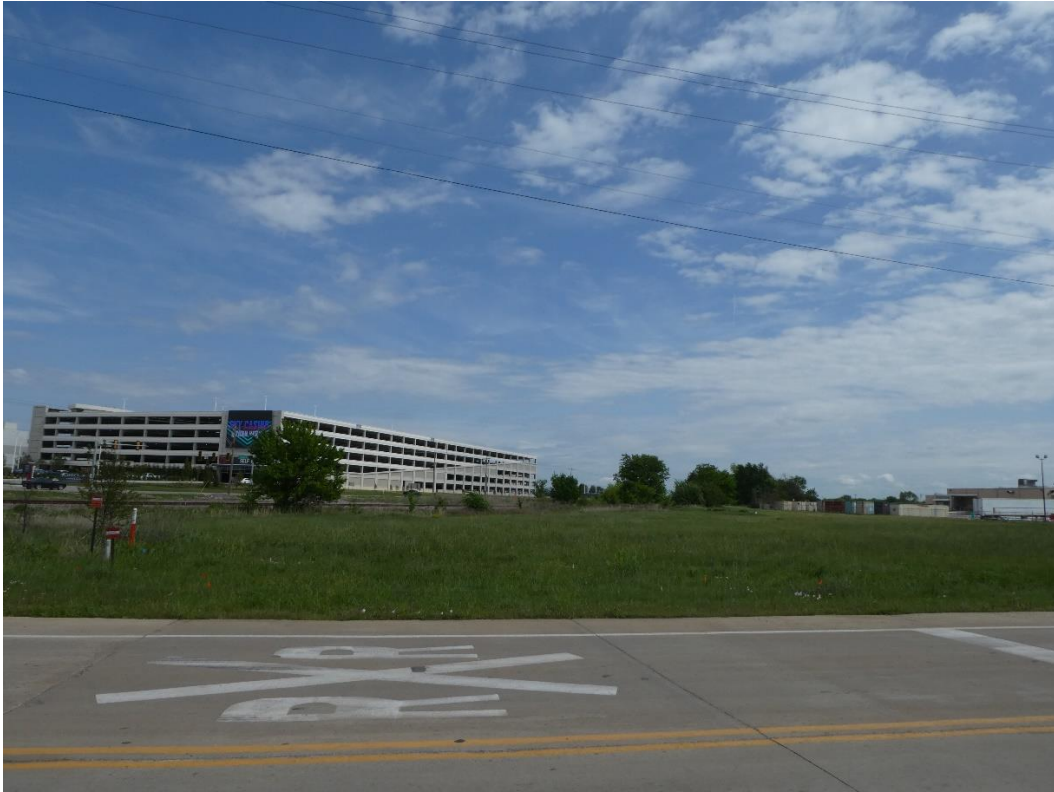
Subject Property – looking north from Waldron Road
